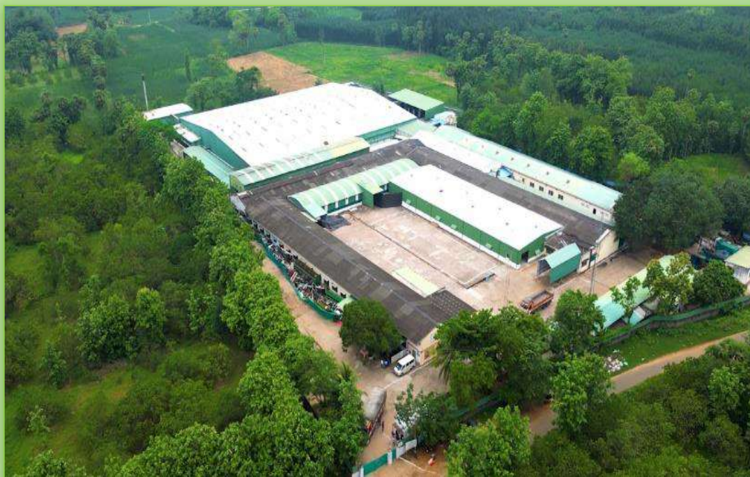
Cashew Processing Plant
